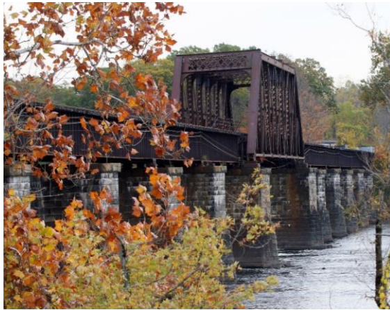
PC: James Roche, Jr. Railroad Bridge over the River
